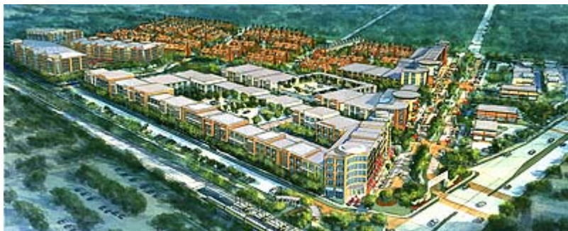
Located in Dallas-Ft. Worth's Telecom Corridor, mixed-use transit-oriented development Brick Row is adjacent to the Spring Valley DART light-rail station. Photo credit: Winston Capital
